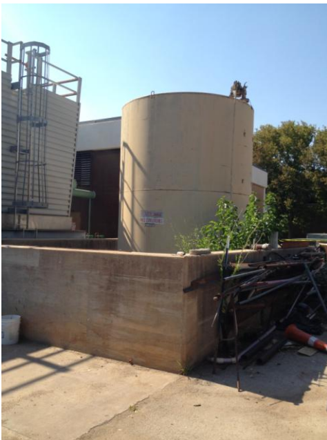
10,000-gallon diesel AST at the Central Plant
