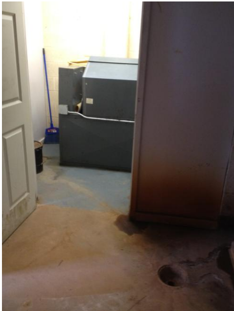
Hardin Administration elevator reservoir with floor drain outside doorway
