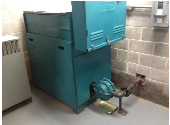
Foster Science elevator reservoir
