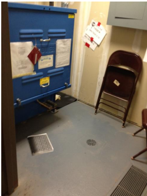
Chapel on the Hill elevator reservoir with floor drain and air vent
