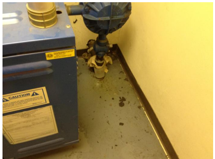
McGlothlin Campus Center Book Store elevator reservoir with leak
